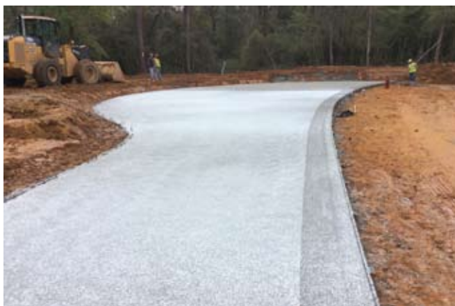
Completed concrete pour for a drive lane at Black Oak
